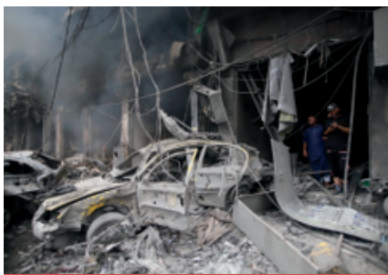
DAMAGE FROM AN ISRAELI AIRSTRIKE IN GAZA
